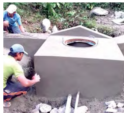
Construction of Interruption Chamber
