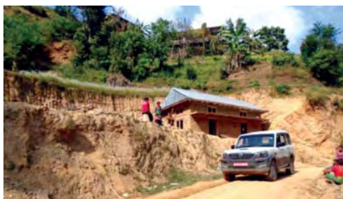
A vehicle in the motor road constructed
