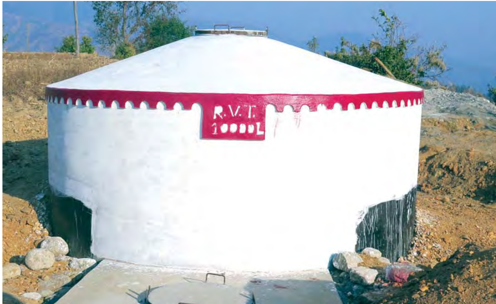
Reservoir tank at Ghokshila
