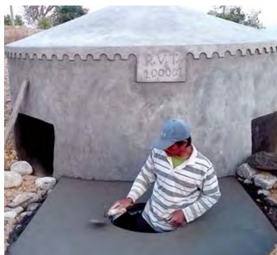
Locals constructing reservoir tanks
