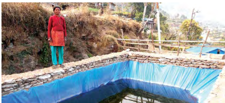
Mrs. Laxmi besides the rainwater harvesting plastic pond used to collect water for vegetable farming.
