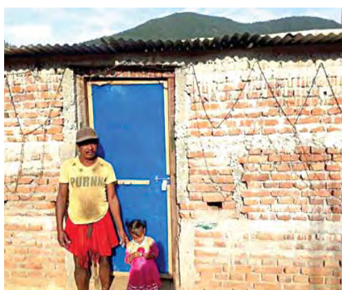
Mr. Bhami Majhi in front of his house being constructed
