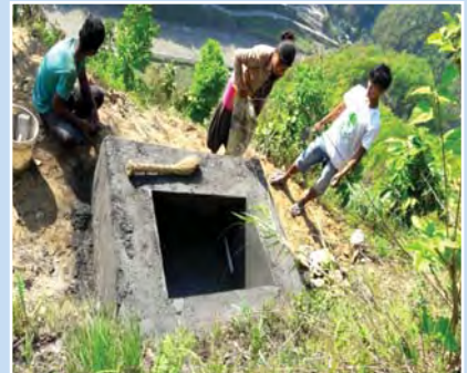
A structure to break water pressure being constructed
