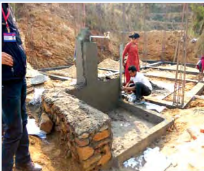
Community members constructing tap stand
