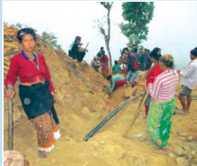
Locals digging a trench to put in water distribution pipe line
