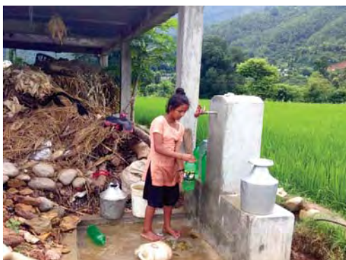
A girl collecting water in CN constructed tap stand
