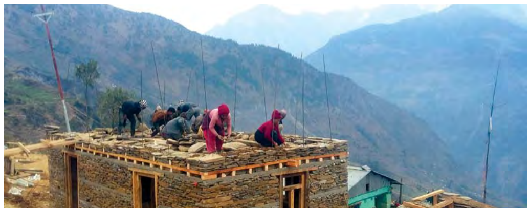
Swostika Khatri constructing a house in Orang (Bigu-2)
