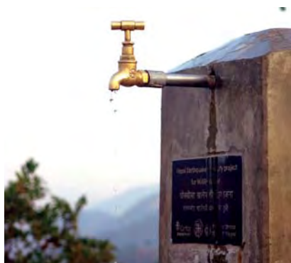
A tap stand constructed
