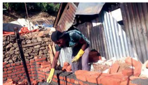
Mr. Sundar Pahari busy constructing shelter in Pahari settlement
