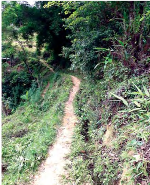
Road before CN's intervention
