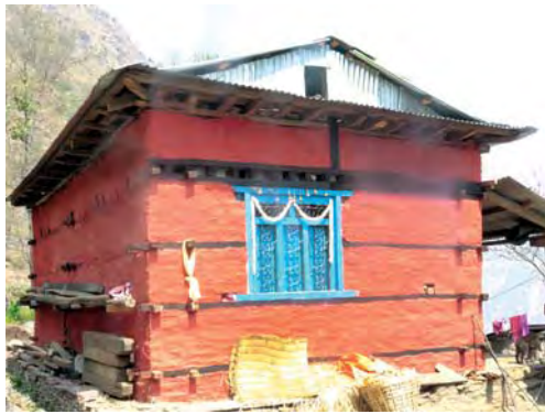
Master Sanjay Tamang's stone mud masonry house with wooden bands.
