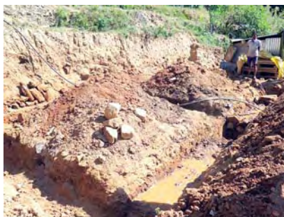
Water being used for shelter construction
