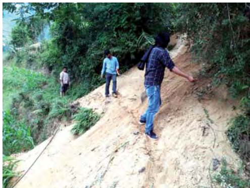
CN's technicians undertaking a survey of the road
